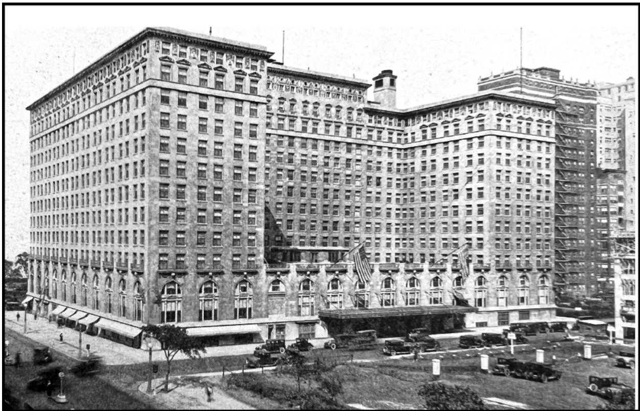
The Drake Hotel as the Fostoria High School Band would have seen it. Note the old cars in the photo.
